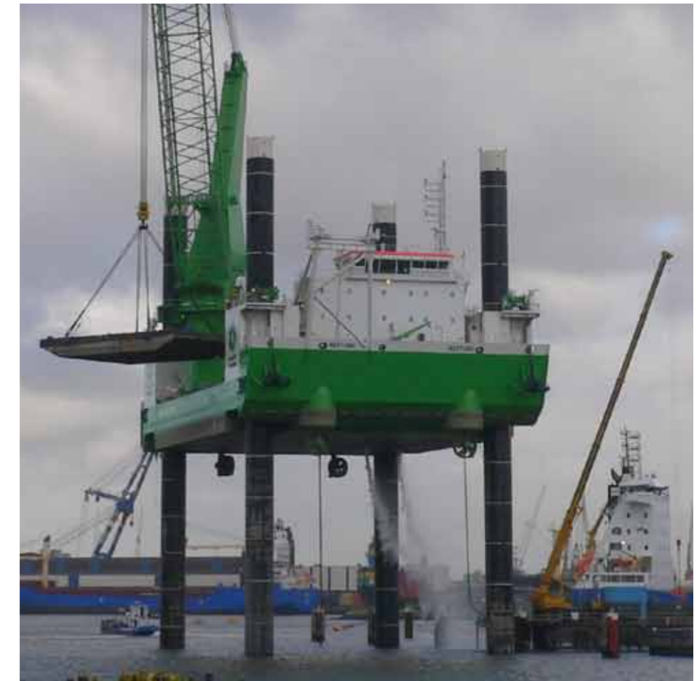
Deepwell pumps provide the cooling water through flexible hoses when jacked-up
