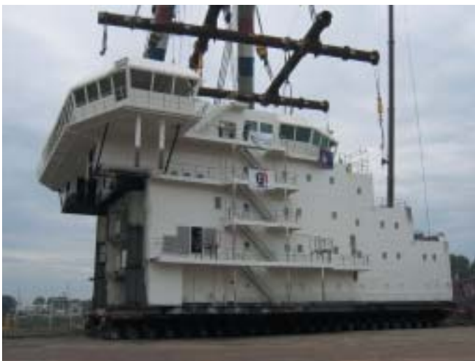
*The superstructure was placed after the launching of the hull
