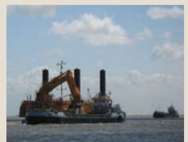
and excavator dredgers
