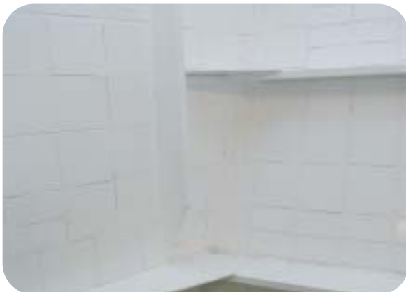
The bulkheads of the tunnel thruster room received a visco-elastic damping treatment to reduce the noise
